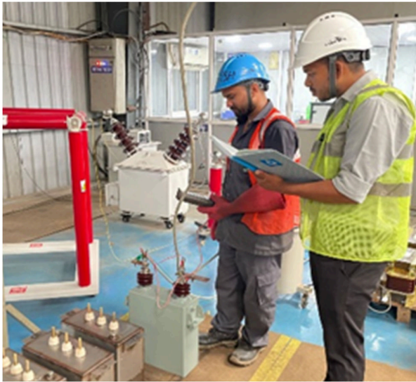
Capacitor HV testing
