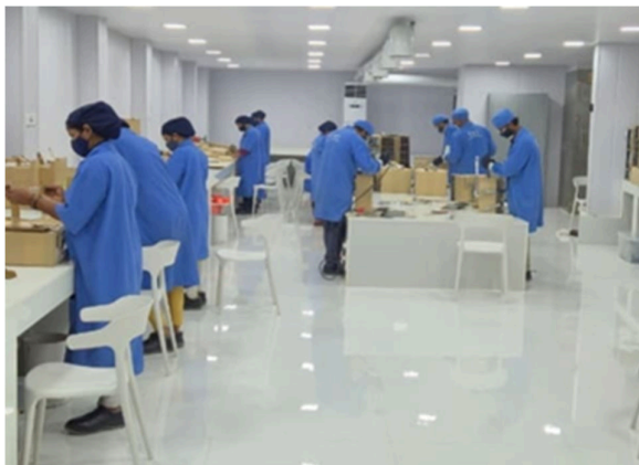
Dry Assembly of Clean room
