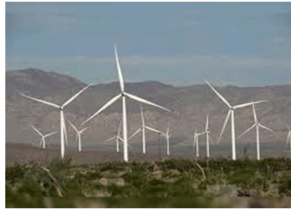
Wind Farm Power Plant
