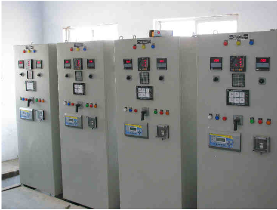
CONTROL & RELAY PANELS
