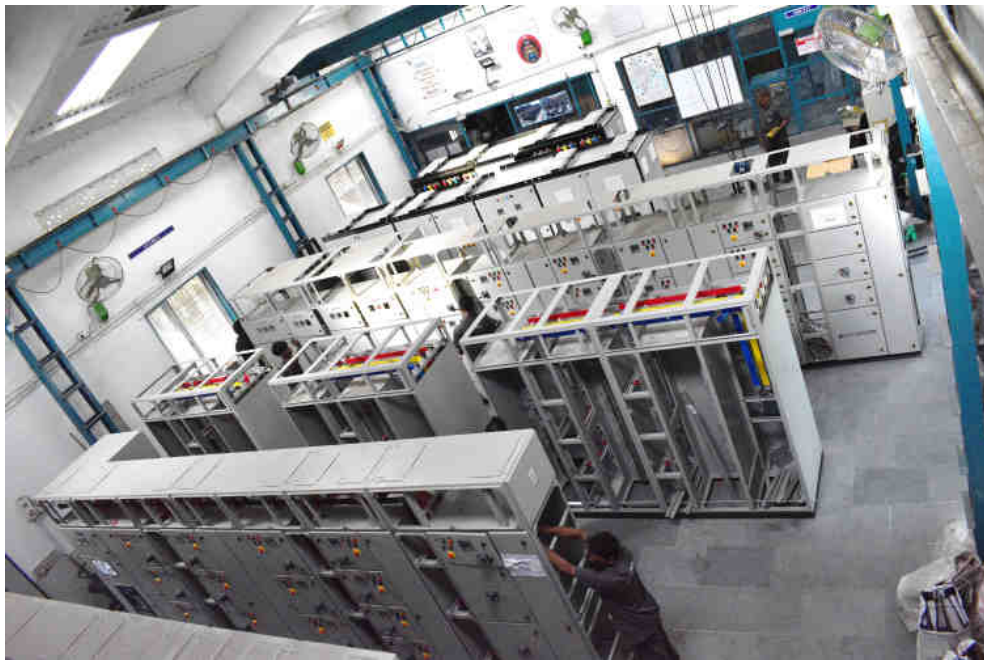
BIRD'S EYE VIEW OF THE ASSEMBLY AREA
