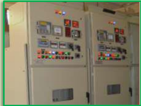
Indoor MV Switchgears upto 33 kV
