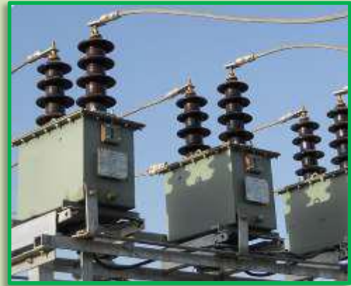
MV Current and Voltage Transformer upto 33 kV
